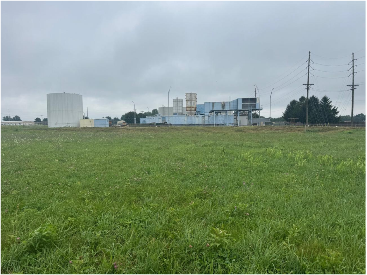
View toward adjacent IMU Facility to South.
