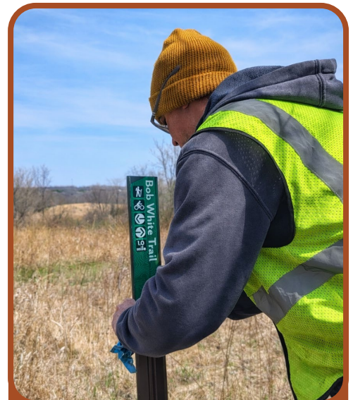
Installing Signpost, Central City Iowa. Image: Backyard Trails LLC
