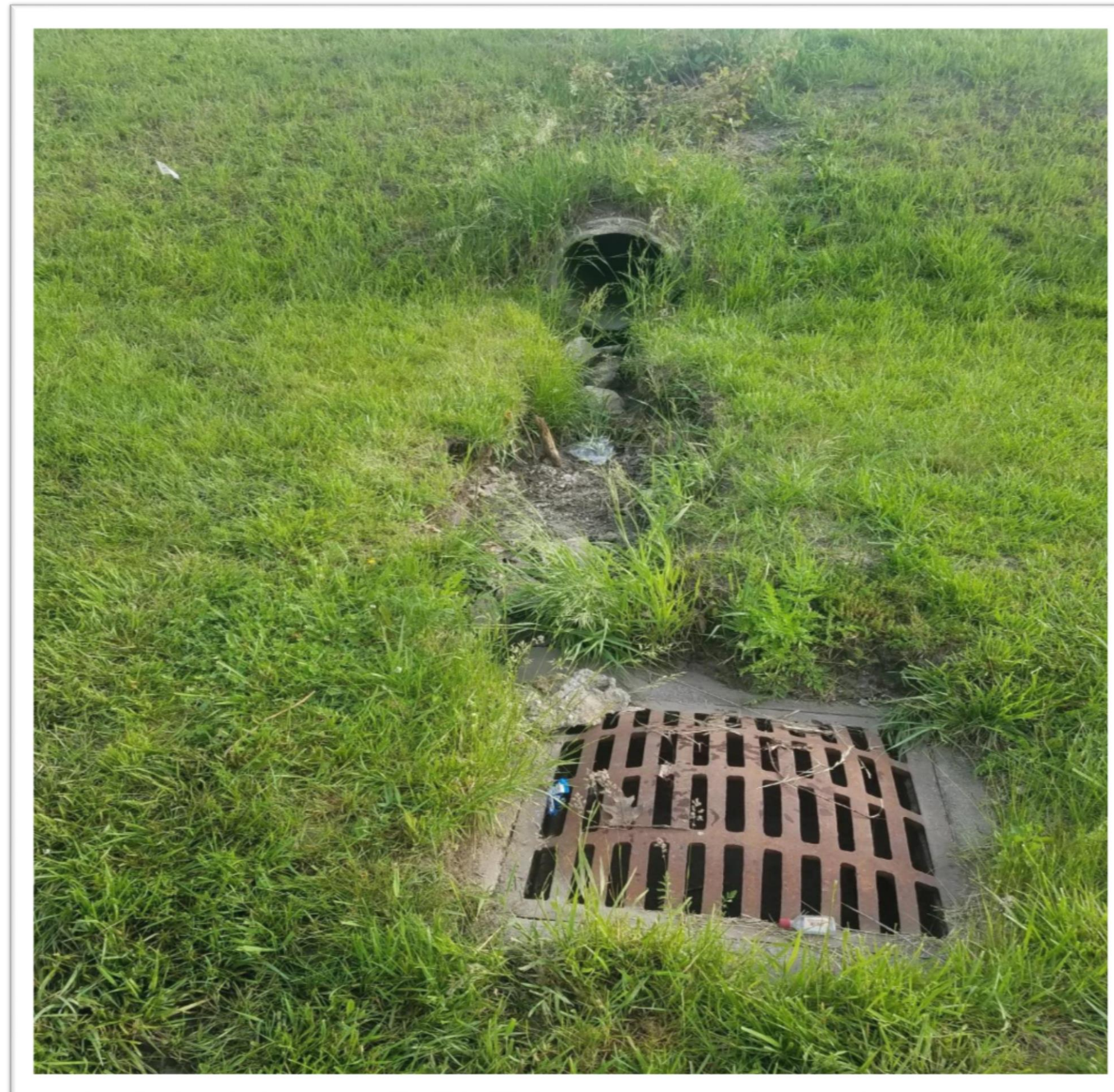
Hillcrest Avenue Culvert- Before/After pics
