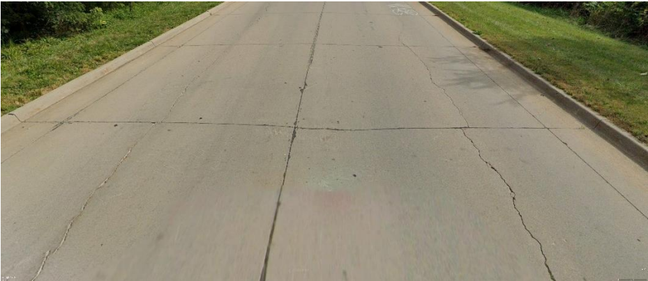
FIGURE 11: EXAMPLE OF “GOOD” CONDITION PCC – W IOWA AVENUE W Iowa Avenue, west of N L Street, has a CityPCI score of 66/100
