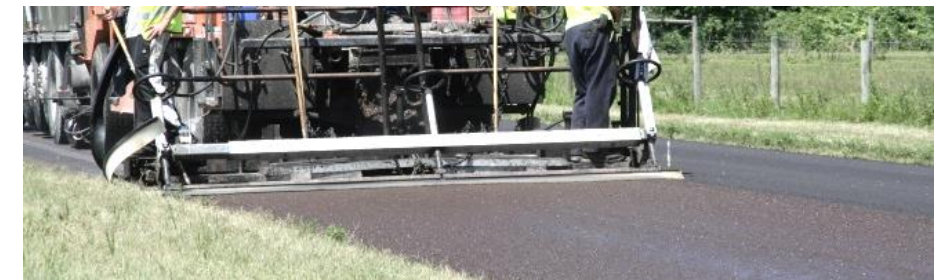
FIGURE 24: MICROSURFACING CREW AT WORK (ERIC PULLEY)
