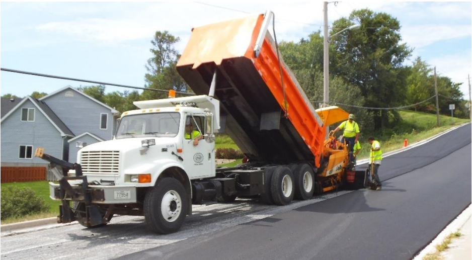
FIGURE 20: HMA OVERLAY ON MILLED PAVEMENT (COUNCIL BLUFFS) This is a picture of an asphalt overlay placed in the City of Council Bluffs following milling of the existing pavement surface.
