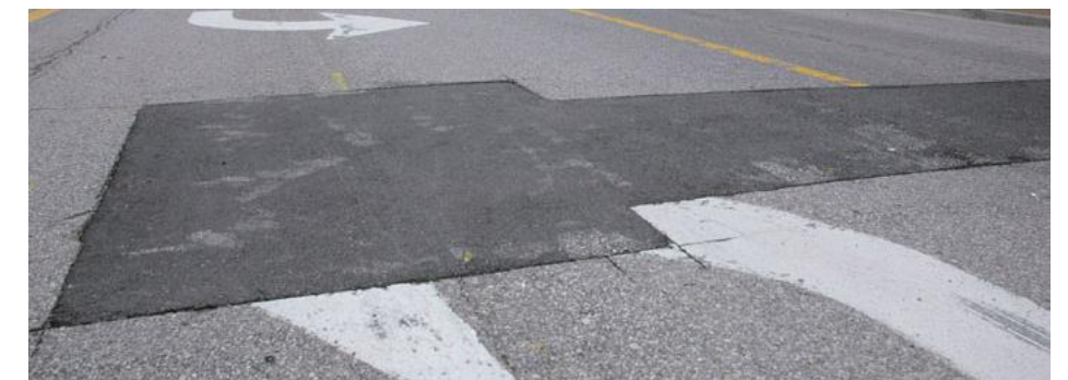
FIGURE 25: HMA PATCHING WITH LOCALIZED PAVEMENT REMOVAL
