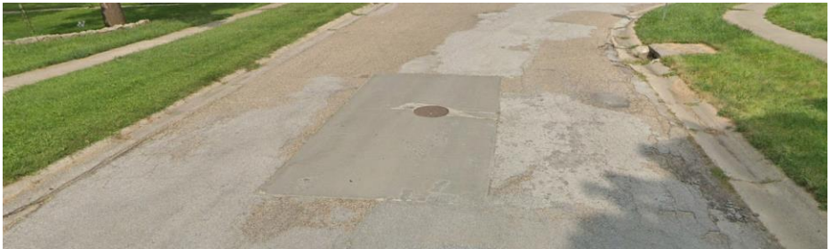
FIGURE 14: EXAMPLE OF “POOR” CONDITION COM – W LINCOLN AVE W Lincoln Avenue, just east of N C Street, has a City PCI score of 39/100.
