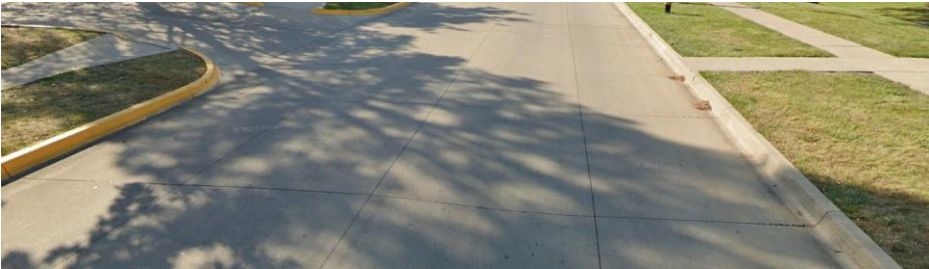
FIGURE 9: EXAMPLE OF “VERY GOOD” CONDITION PCC – N E STREET N E Street, north of Franklin Avenue, has a CityPCI score of 92/100
