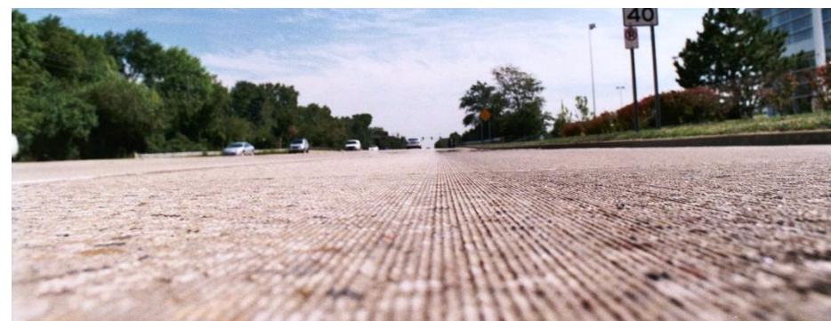
FIGURE 23: PAVEMENT AFTER DIAMOND GRINDING (JOHN ROBERTS)
