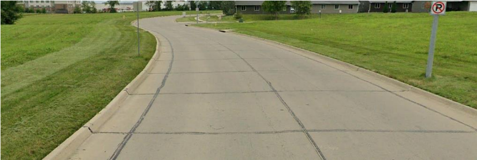
FIGURE 10: EXAMPLE OF “VERY GOOD” CONDITION PCC – N 9 TH STREET N 9 th street, north of E Madison Avenue, has a CityPCI score of 89/100
