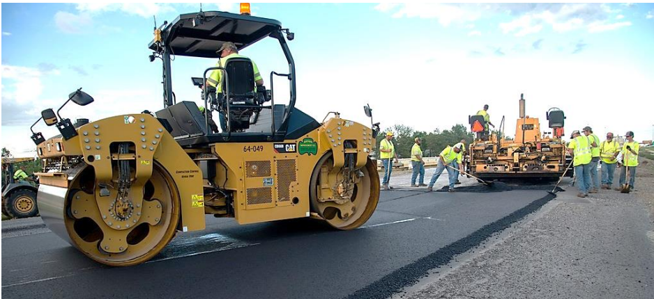
FIGURE 19: RECONSTRUCTION OF I-94 (NDDOT) This photo shows the Construction of a-new asphalt cement concrete pavement
