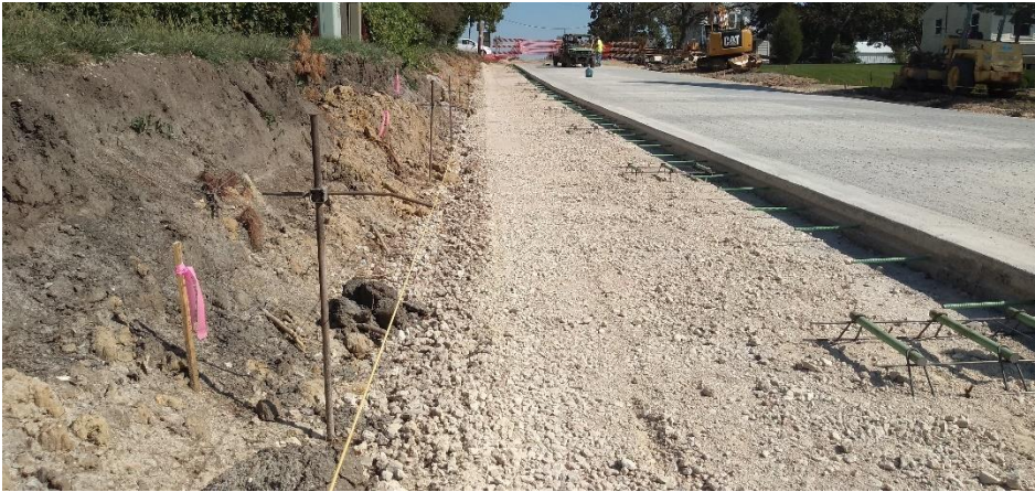
FIGURE 18: PCC RECONSTRUCTION OF DIVISION STREET This photo shows a road during a PCC reconstruction project located in Swisher, IA.
