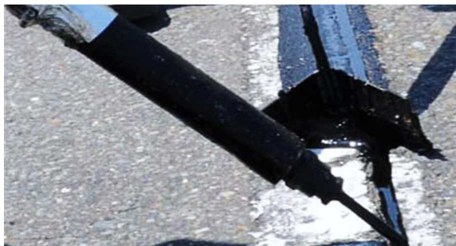
FIGURE 22: CRACK SEALING PERFORMED W/ ROUTING (USAF)
