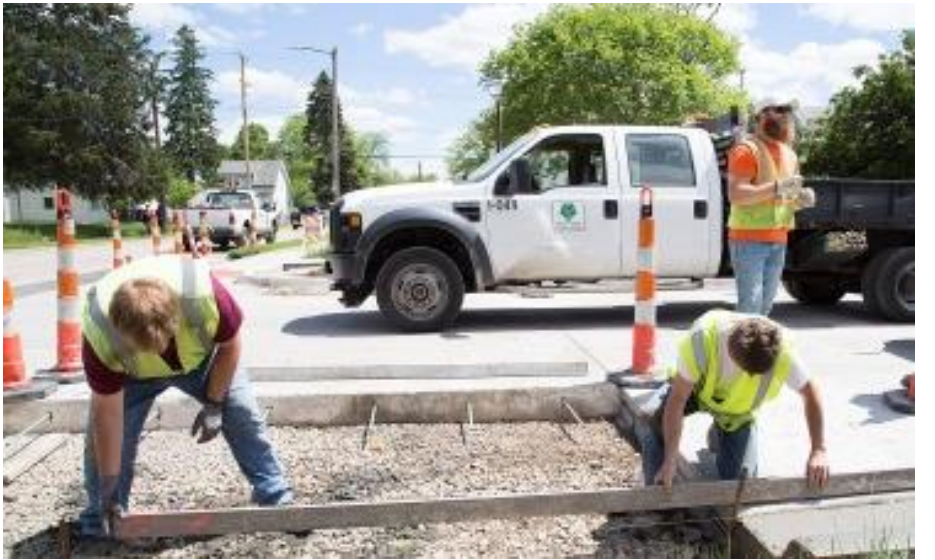
FIGURE 21: PCC RESTORATION (CITY OF CEDAR RAPIDS). This is a picture of a city maintenance crew in Cedar Rapids performing a panel replacement as part of a larger concrete restoration project.
