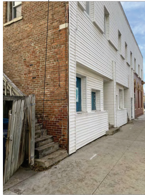
EXISTING PHOTOGRAPH EXISTING IMAGE OF SOUTH SIDE OF FACADE
