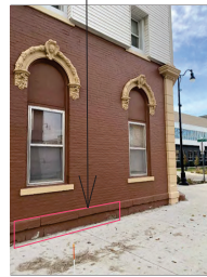
EXIST. PHOTO EXISTING IMAGE OF NORTH WINDOWS W/ WOOD FILL IN
