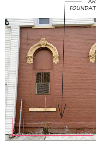
EXIST. PHOTO EXISTING IMAGE OF SOUTH WINDOW W/ A/C & WOOD FILL IN
