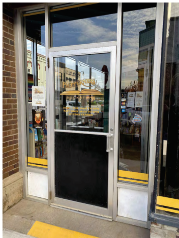
EXISTING PHOTOGRAPH EXISTING IMAGE OF "NORTH" ENTRANCE STOREFRONT SYSTEM THAT IS BEING REPLACED
