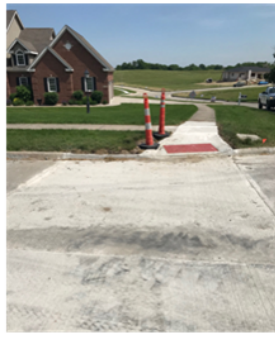
The above pictures shows the repairs of the deteriorated concrete pavement sections and the upgrades to ADA compatible sidewalk ramps on the cul-de-sac of Sunset Circle.
