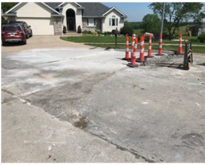
The above pictures shows the repairs of the deteriorated concrete pavement sections and the upgrades to ADA compatible sidewalk ramps on the cul-de-sac of Sunset Circle.
