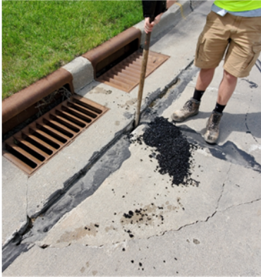
The above pictures shows the before-after repairs of the failed stormwater intake on North U Street.
