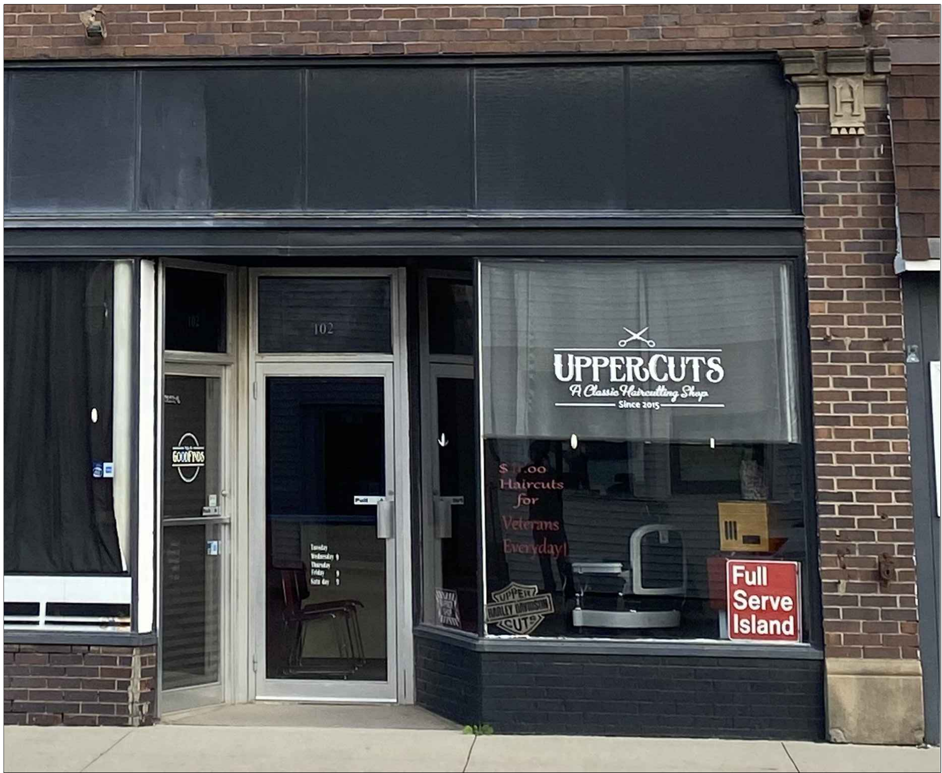
EXISTING PHOTOGRAPH EXISTING IMAGE OF "SOUTH" ENTRANCE STOREFRONT SYSTEM THAT IS BEING REPLACED
