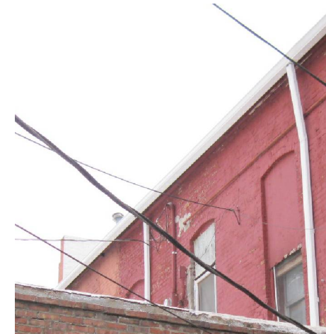
NORTH OUTSIDE WALL SECOND FLOOR VIEW LOOKING SOUTH
