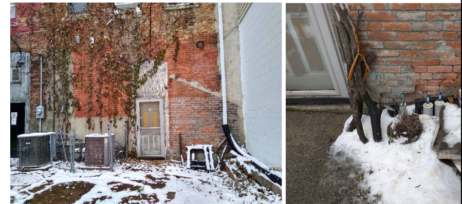
NORTH OUTSIDE WALL VIEW LOOKING SOUTH
