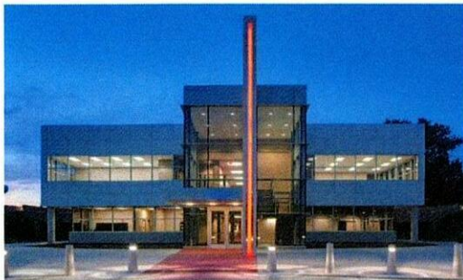
Existing Main Entrance
