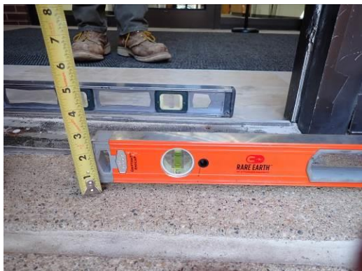
93, 94. Sloping concrete at entry
