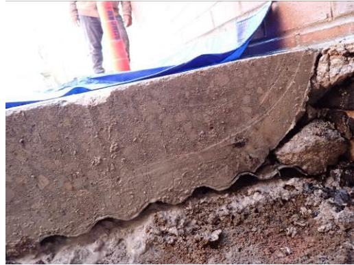
97, 98. Close up views, galvanized "steel centering" supporting concrete
