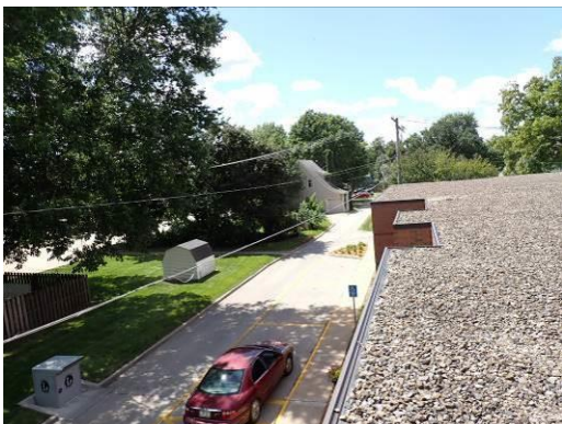
47, 48. Additional views of roof
