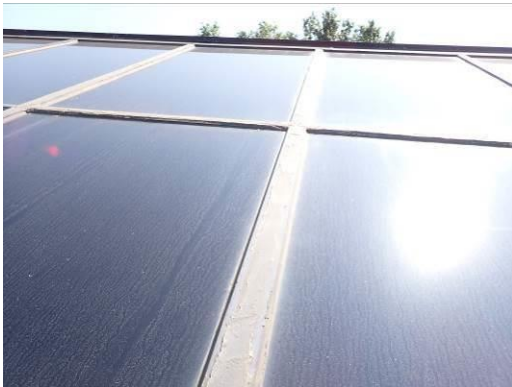
51, 52. Views of repairs to skylights
