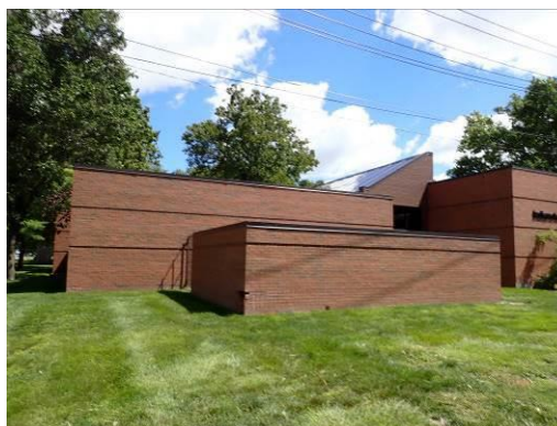
2. View from the southwest
