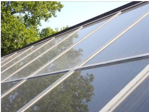
53, 54. Views of skylights
