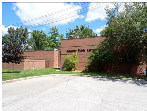
1. View from the west
