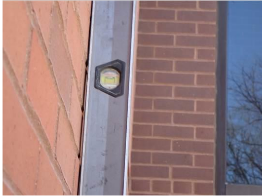
105, 106. Leaning wall, outside alignment
