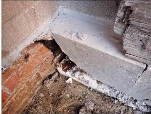
97, 98. Close up views, galvanized "steel centering" supporting concrete
