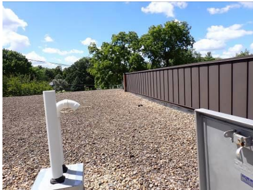
37, 38. Views of roof
