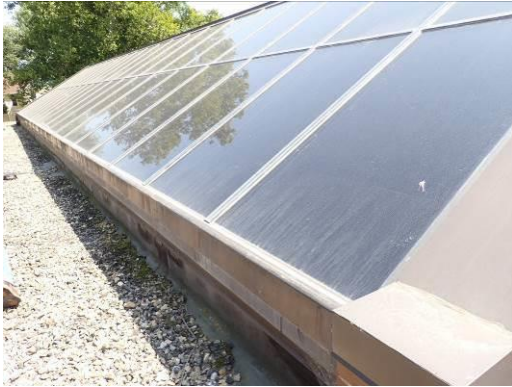
49, 50. Views of skylights
