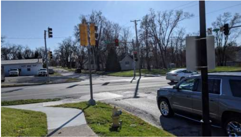
Photo 2. Iowa Highway 92 & Buxton Street (New Curb Ramps)
