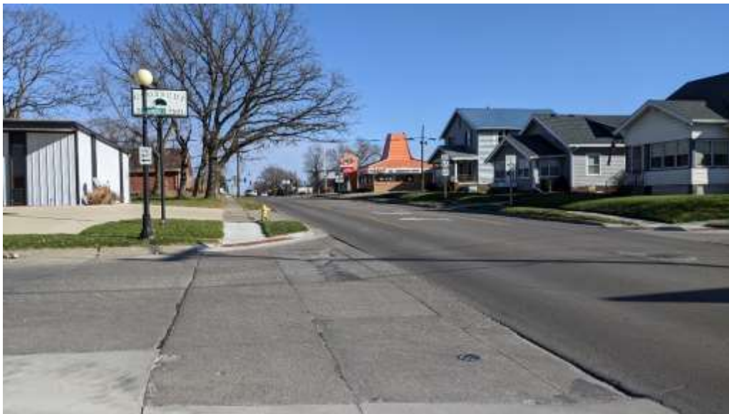
Photo 3. Iowa Highway 92 & Howard Street (New Curb Ramps)
