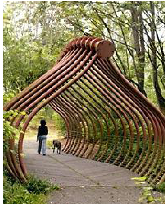
Salmon Bond Bridge
