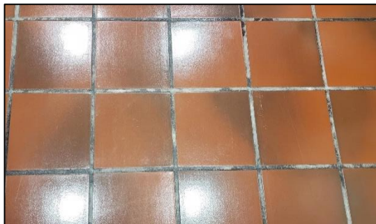
Entryway tile (installed in 1984)
