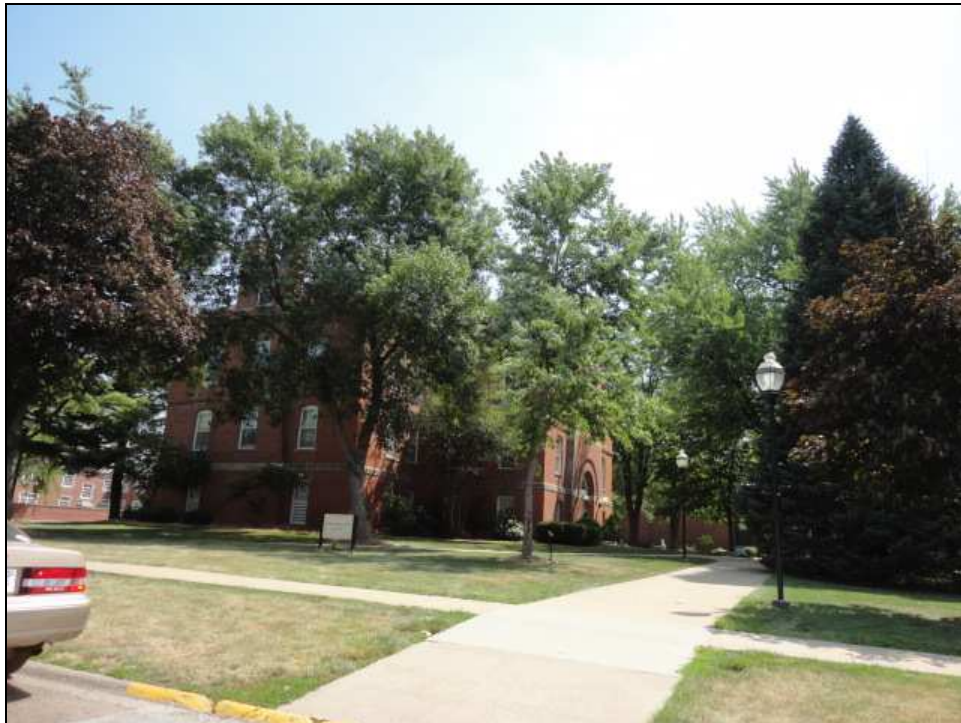
Adjoining Property to the East
