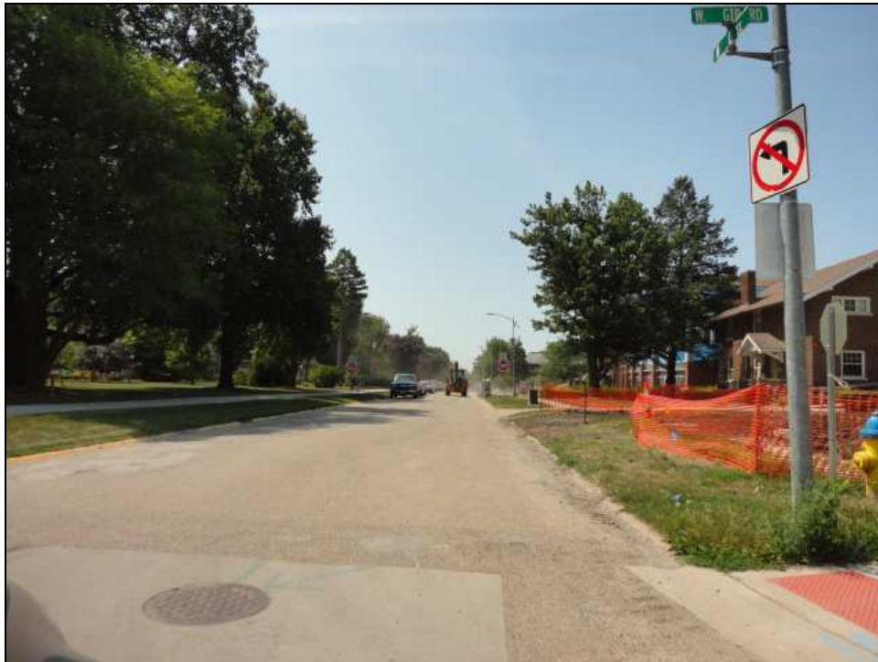
Looking South at Subject
