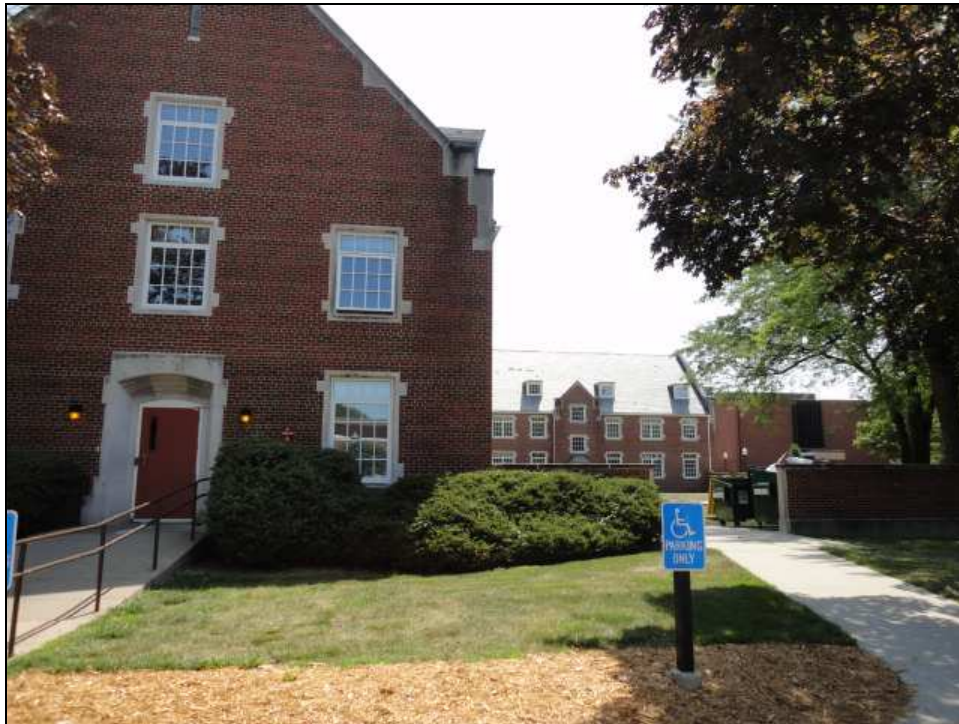
Adjoining Property to the East
