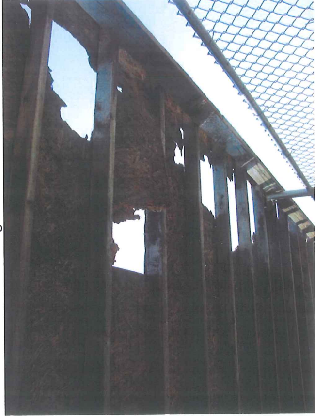
Dug Out Roof
