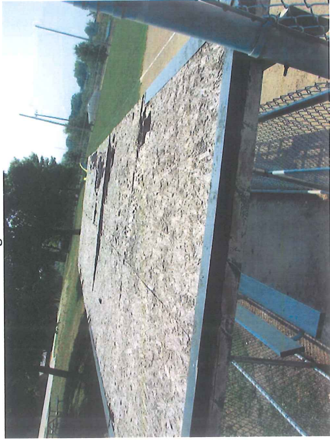
Dug Out Roof
