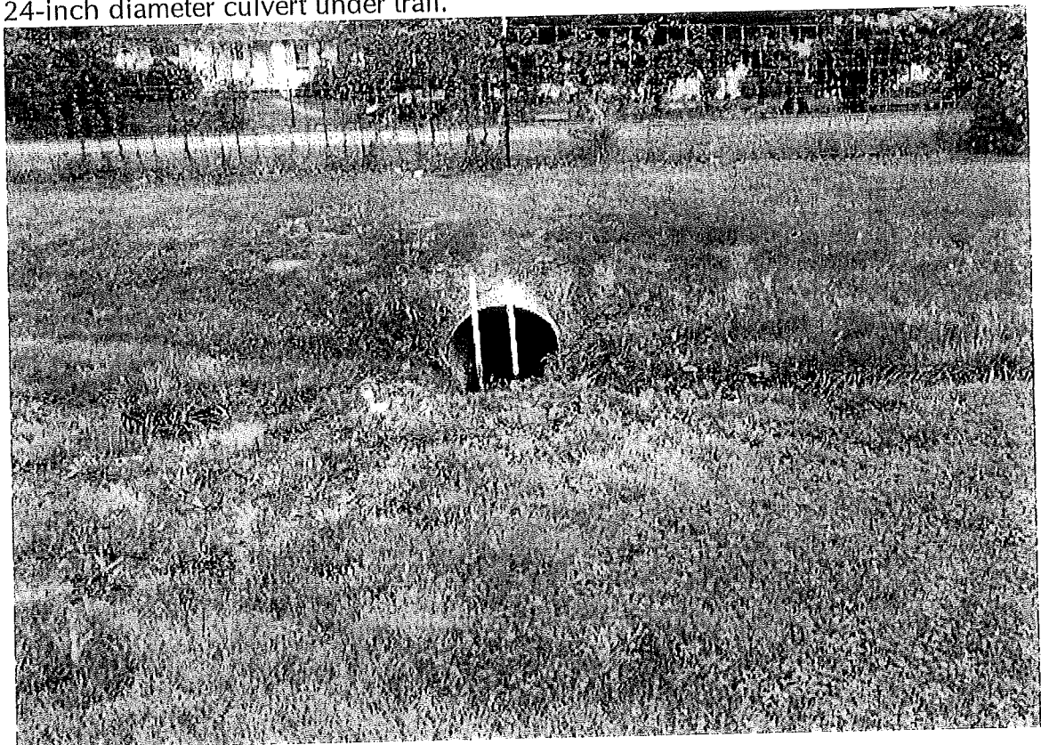
24-inch diameter culvert under trail.
