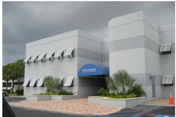
Palm Beach County Water Utilities
