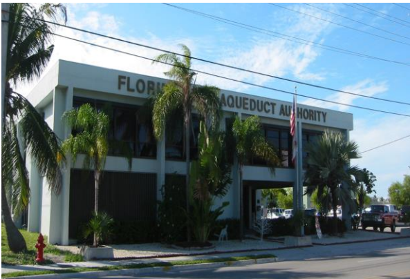
Florida Keys Aqueduct Authority (provides water and some sewer service to the Florida Keys)
